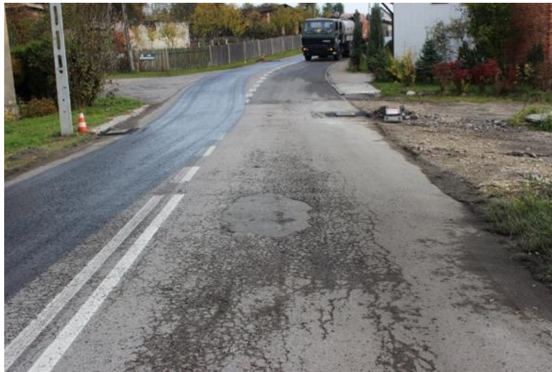
Initial pavement condition - 2013
