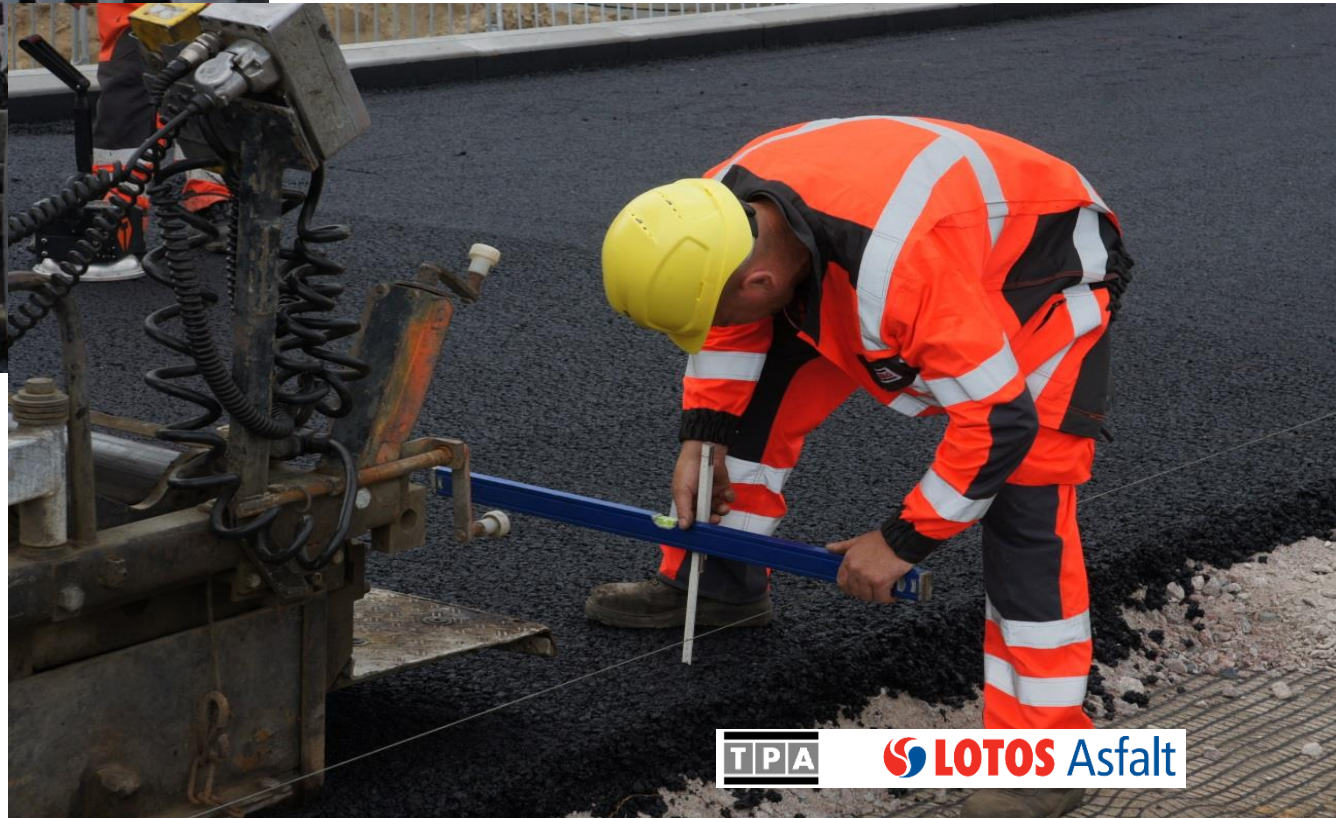
Fig 1., Fig.2. Paving of SMA 16 PMB 45/80-80 anti-fatigue base course
