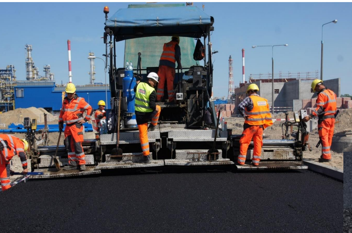
Fig 5. Paving of SMA 22 PMB 25/55-80
