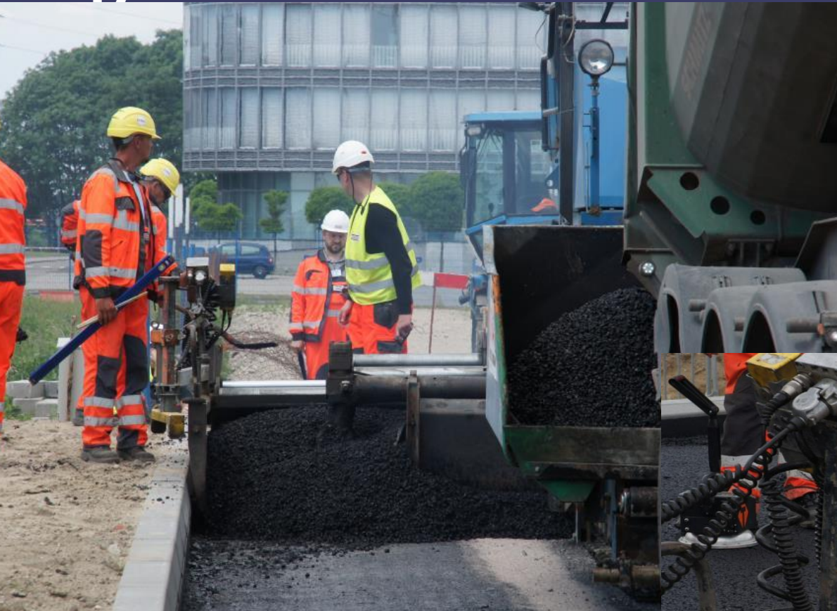
Fig 1., Fig.2. Paving of SMA 16 PMB 45/80-80 anti-fatigue base course
