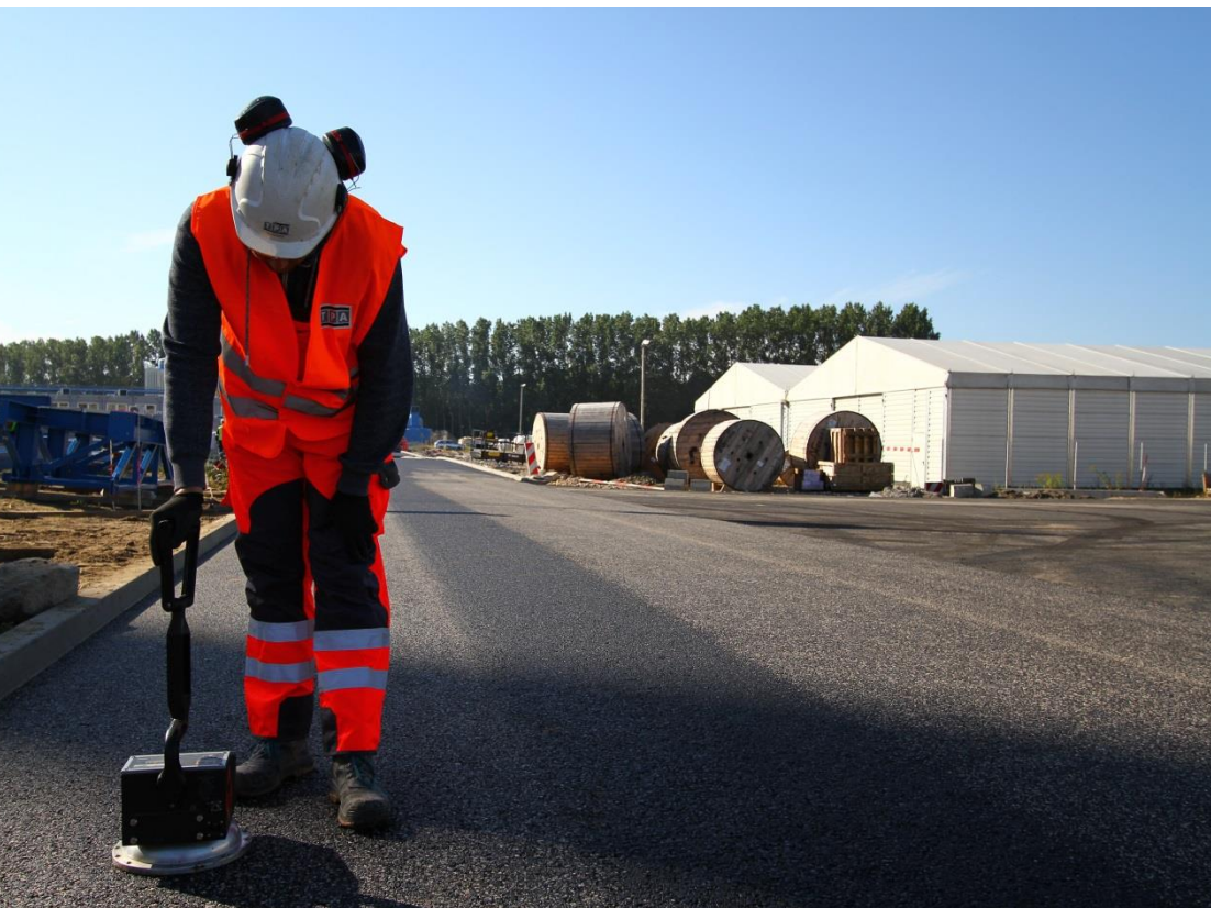
Fig 3. Paving control on site by using PQI sonde
