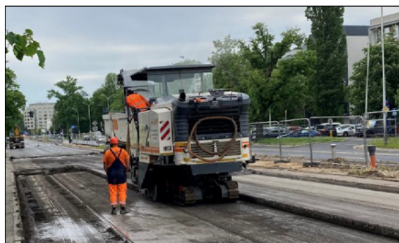
Figure 1. Milling an asphalt pavement – selective milling of individual courses [source: P.Ostrowski]
