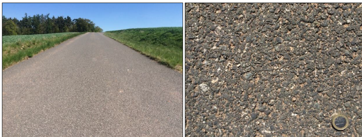
Figure 3: The paved ecycled material after 8 years in May 2025. Scale coin: 1 euro = 23.35mm
